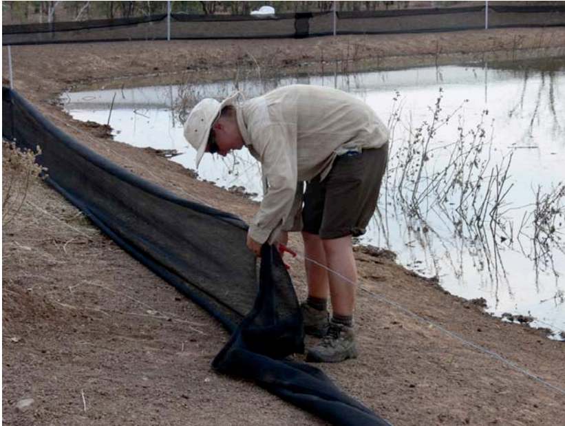
Picture – Volunteer helping to erect the fence.
